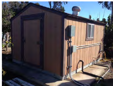
B. Plover shed was installed atop a concrete slab that formerly supported an old cabin
