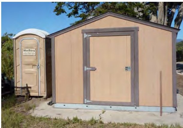
F. Porta-potty Garden shed. Shed was installed atop a concrete slab that formerly supported an old cabin.
